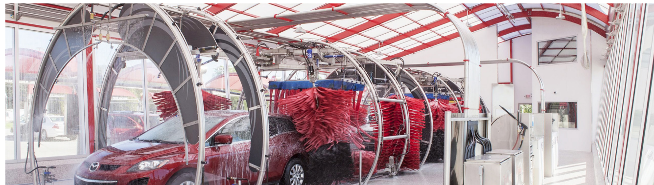
Trusscore Wall&CeilingBoard & NorLock by Trusscore in Commercial Carwash
