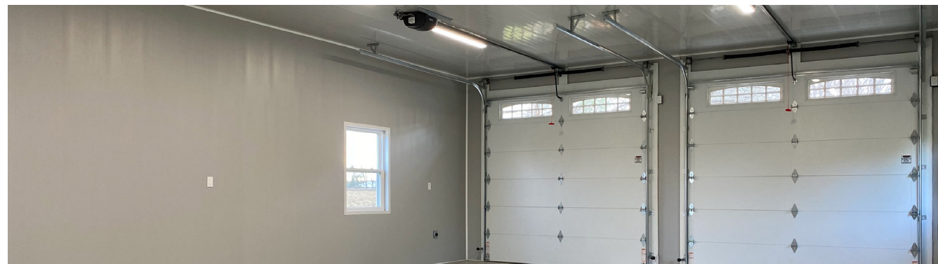
Trusscore Wall&CeilingBoard in Residential Garage
